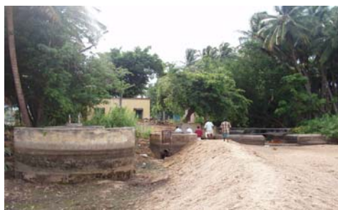
Infiltration well at river Surulivar
