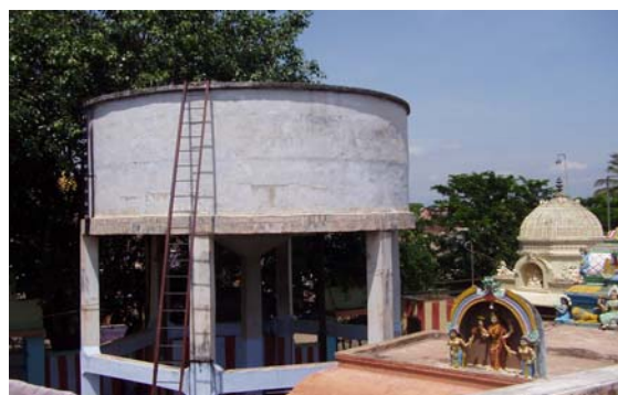
OHT at Samadharamapuram
