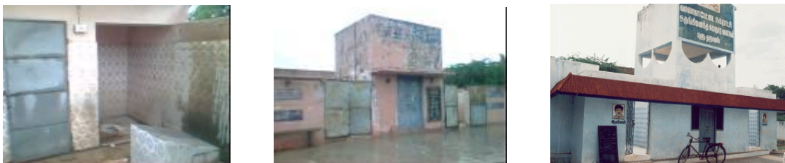
Existing public toilets
