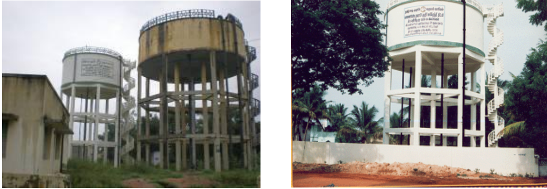
Existing Over Head Tanks
