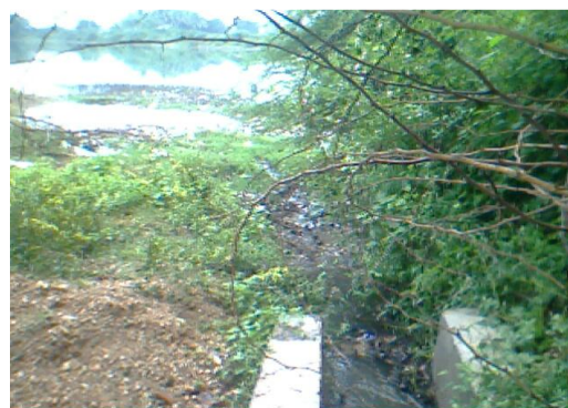
Storm water stagnation area
