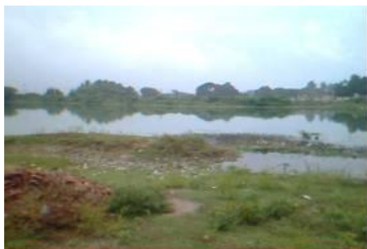
Existing storm water drain
