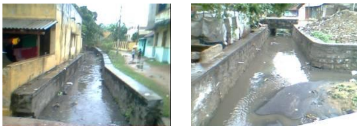
Existing Storm water drains
