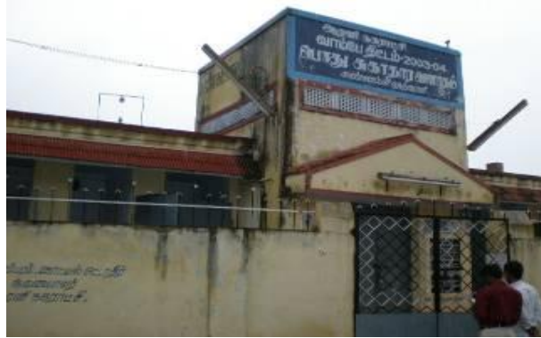
Existing public toilet
