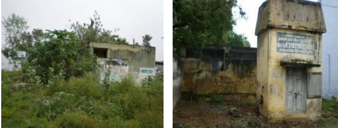
Existing Approach to the public toilets
