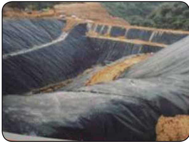
Geotext lining in landfill
