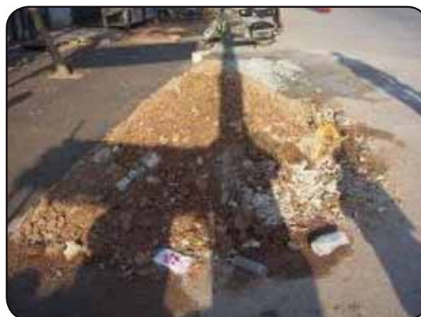
Debris used for repairing the potholes
