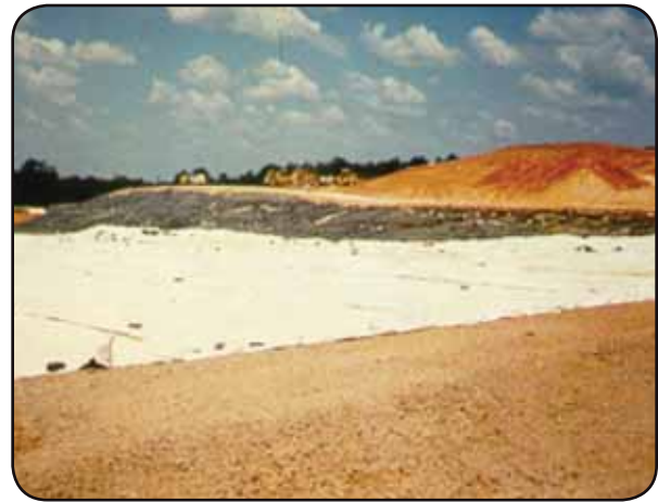
Geotext lining in landfill
