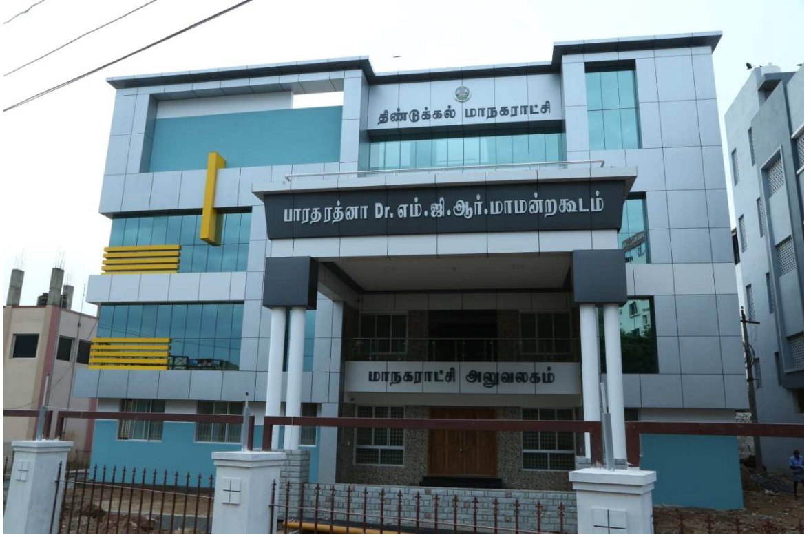
CONSTRUCTION OF NEW OFFICE BUILDING
