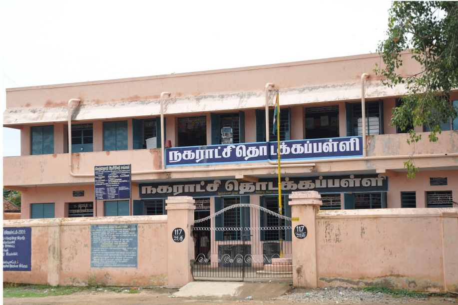
Existing School Building at Thouppukana South Elementary School - Ward No-24
