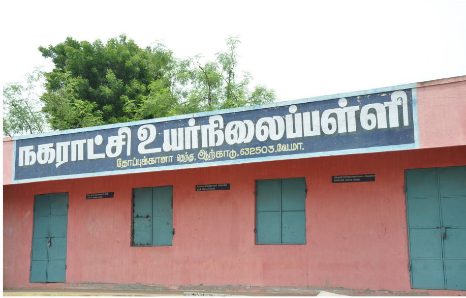
Existing School Building at Thouppukana South High School - Ward No-24
