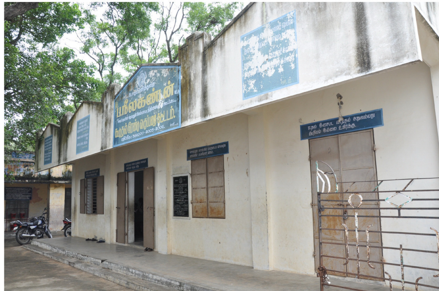
Existing School Building at Anna Nagar Midle School - Ward No-19
