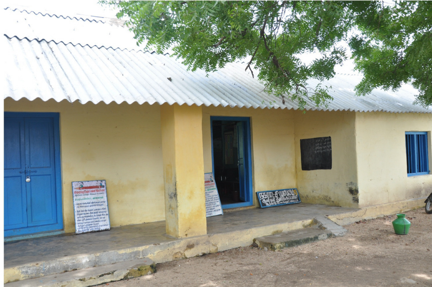
Existing School Building at Y&O Boys Elementary School - Ward No-08
